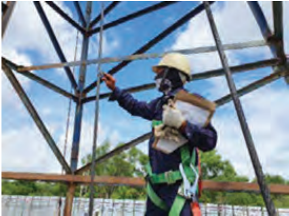
Figure: The contractor's outfit for work at height
