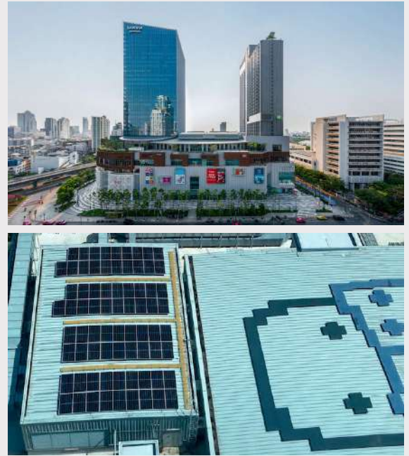
Solar cell installations at Samyan Mitrtown with the capacity of 40 KW
